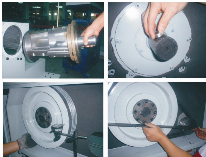
Picture 3-8: Installation of Bearing, Motor, Belt Pulley and Belt
