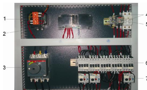
Picture 2-37: Main Electrical Components
